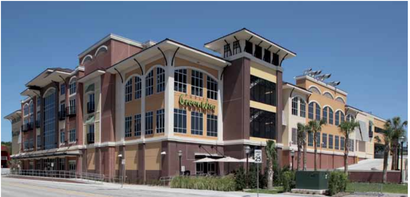
The new GreenWise organic supermarket by Publix Supermarket in Tampa, Fla., combines grocery, retail, offices and parking space in a total precast concrete structural solution that offers the functional needs for each use as well as an attractive façade that fit into the historic neighborhood.
