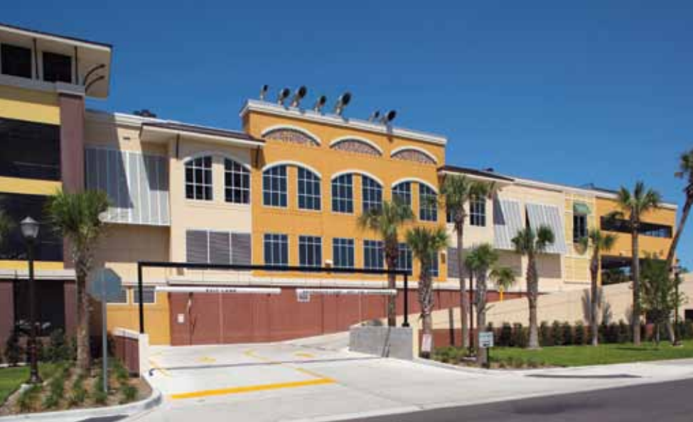
The speed ramp along the back of the building quickly pulls customers up to the parking levels, alleviating congestion on the street. Vent ducts at the top of the parking levels were needed due to the working kitchen and other facilities inside the supermarket on the first floor.
