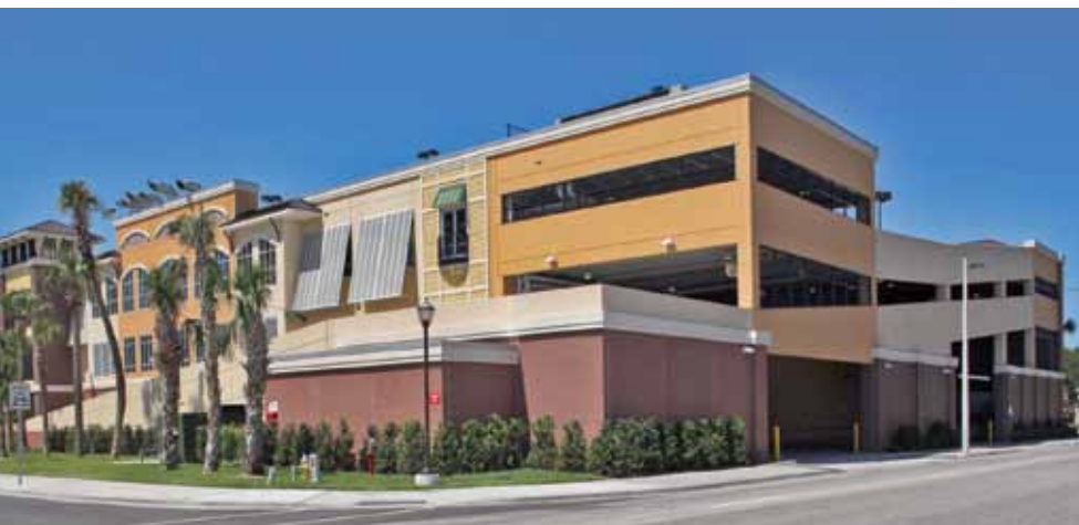
A variety of paint colors and finishes created the appearance of smaller shops along the supermarket and parking facades.
