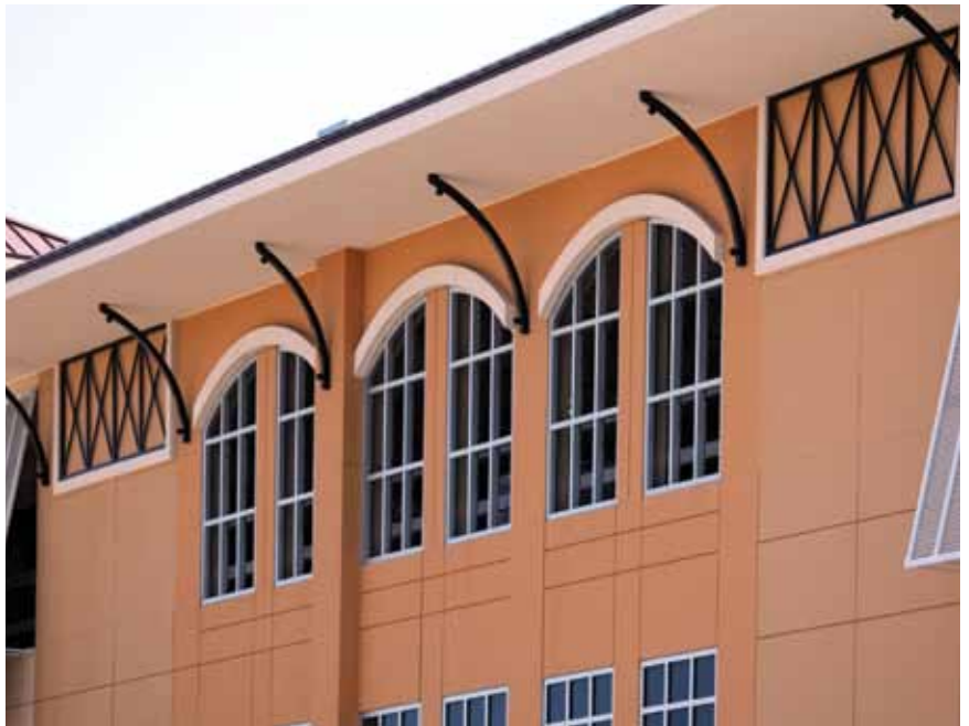
The precast concrete panels were cast with embedded thin brick, cast-in tile mosaics and rustications, with a number of paint colors used. Some were used to create false windows cast into the panels (lower row). These variations were embellished with accessories such as decorative grilles and awnings.
